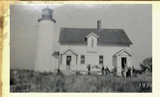
At the time the 2 story house is being built the 39 foot tall light tower under goes modification. It has be raised ten feet higher so it's light will be not be blocked by the new taller house being built next to it. The picture above shows the tower after it has been raised ten feet higher.
